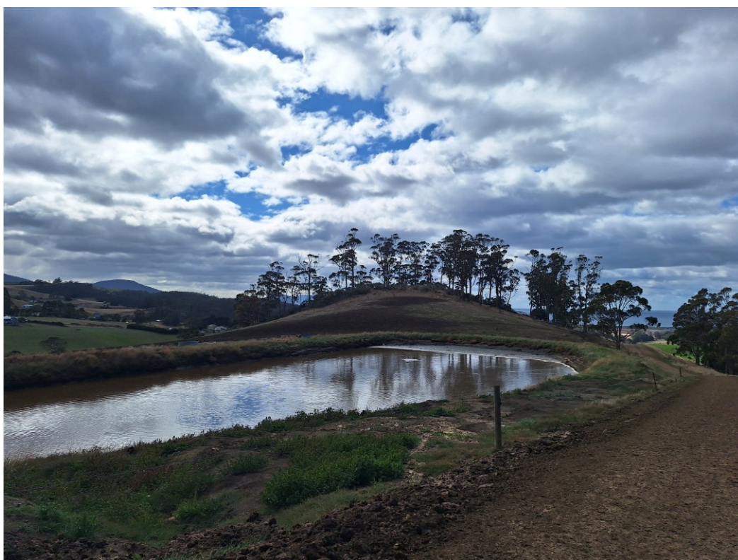
Figure 5 Existing effluent pond
