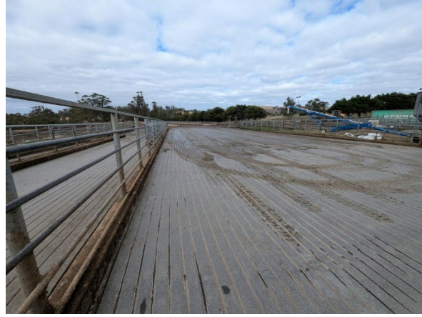
Figure 18. Cow yard after yard blasting the upper part and dry scraping the lower section by front-end loader.
