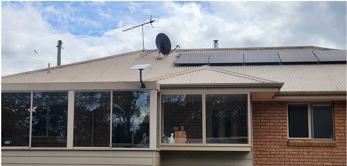
EXISTING ROOF TO CHANGE
