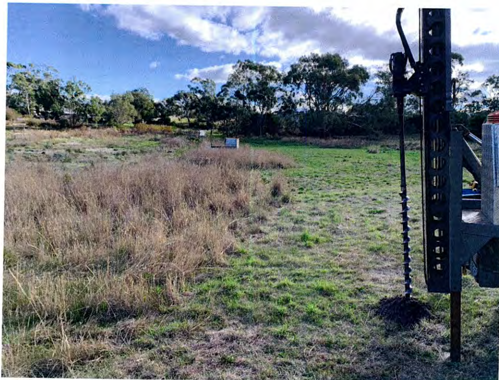
Plate 1 – Test Hole #1 - looking to the north.
