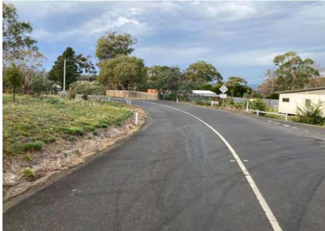
Figure 14 – Carlton River Road Western approach at Gate Five Road
