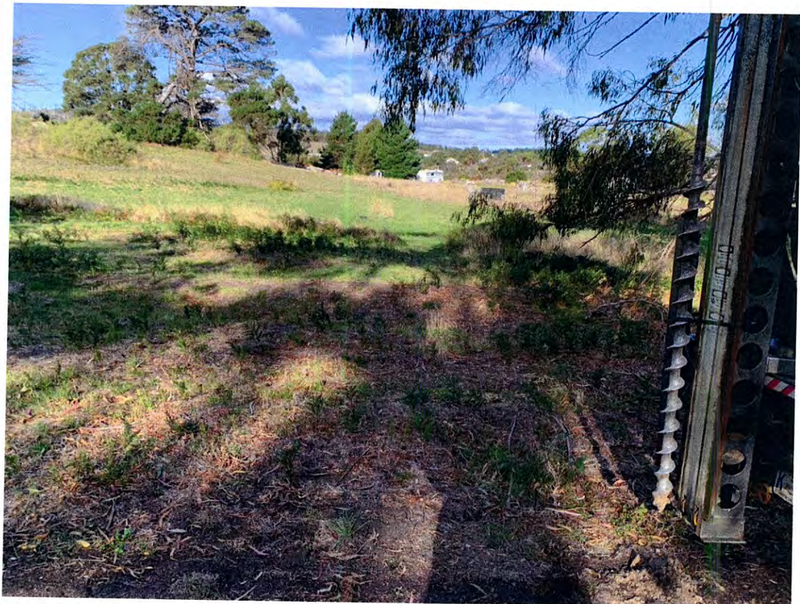
Plate 5 – Test Hole #5 - looking to the southeast.
