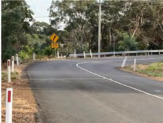
Figure 7 – Carlton River Road Eastern approach to Gate Five Road.
