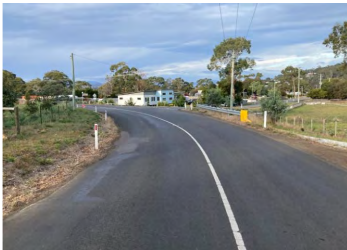
Figure 13 – Carlton River Road Western approach to Gate Five Road
