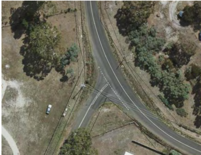
Figure 12 – Aerial view of Carlton River Road / Gate Five Road junction
