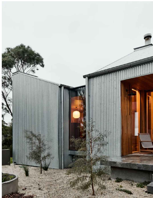
ZINCALUME CUSTOM ORB AND GRAVEL FIRE BREAK
