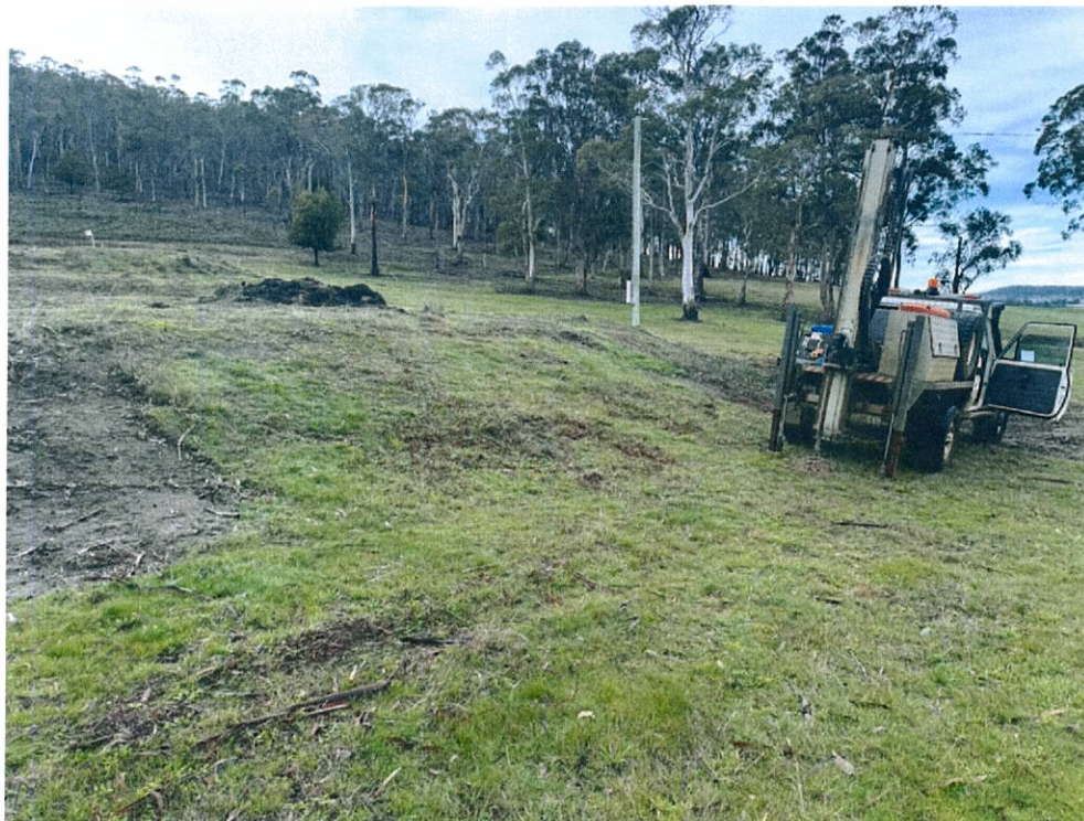
Plate 2 – Test Hole #2 – Immediately downslope from the fill pad - looking to the east/southeast.
