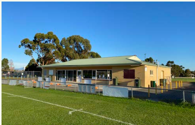
8 Clubhouse with change rooms, toilets and kiosk
