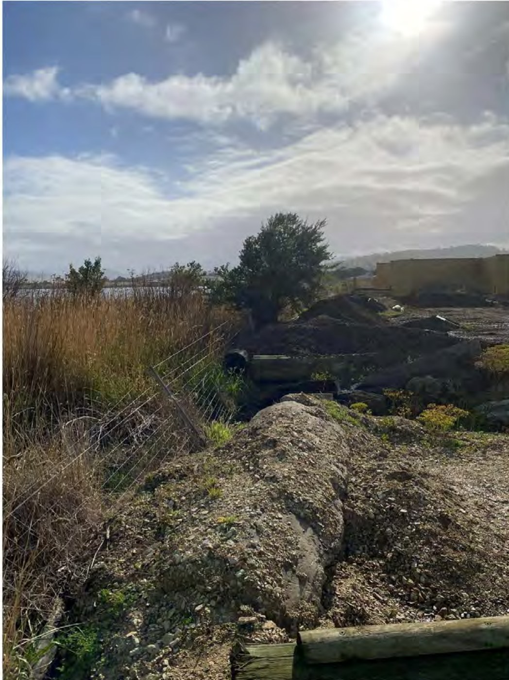
Attachment 1 - 139 Main Rd, Sorell - boundary fence - PWS image 1
