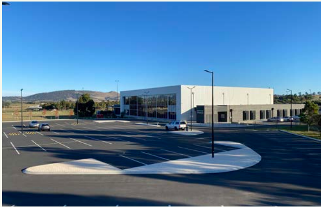
1 South East Stadium and car parking
