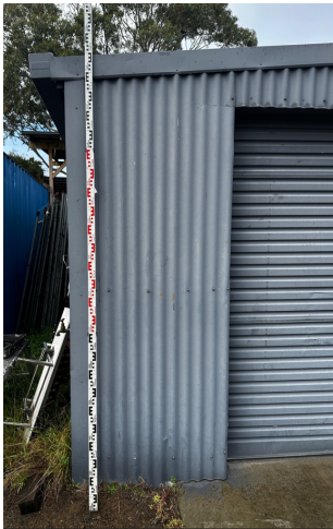
Shed Lean-to 2.5m high (on eave, 2.8m on high side where meeting original shed)
