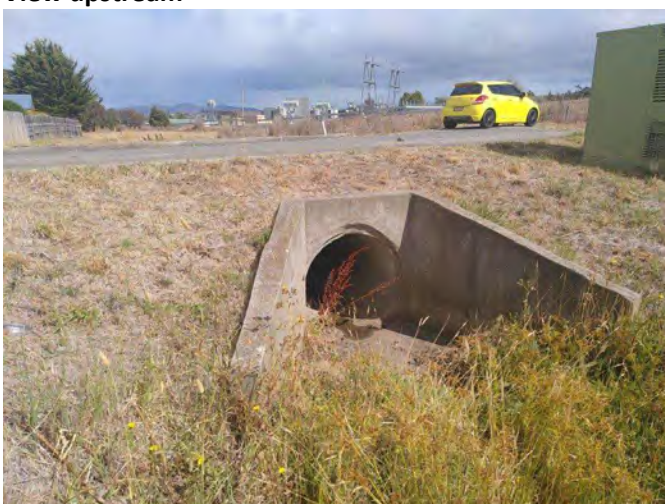
Leitram Avenue culvert
