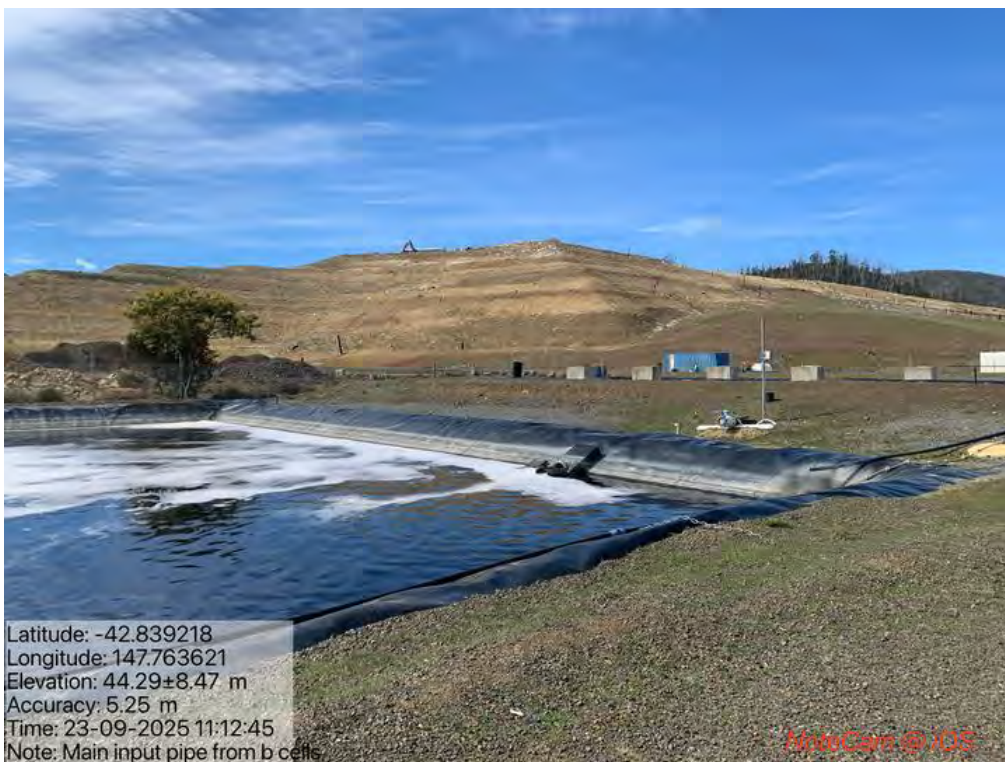
Figure 3 B cell leachate on site
