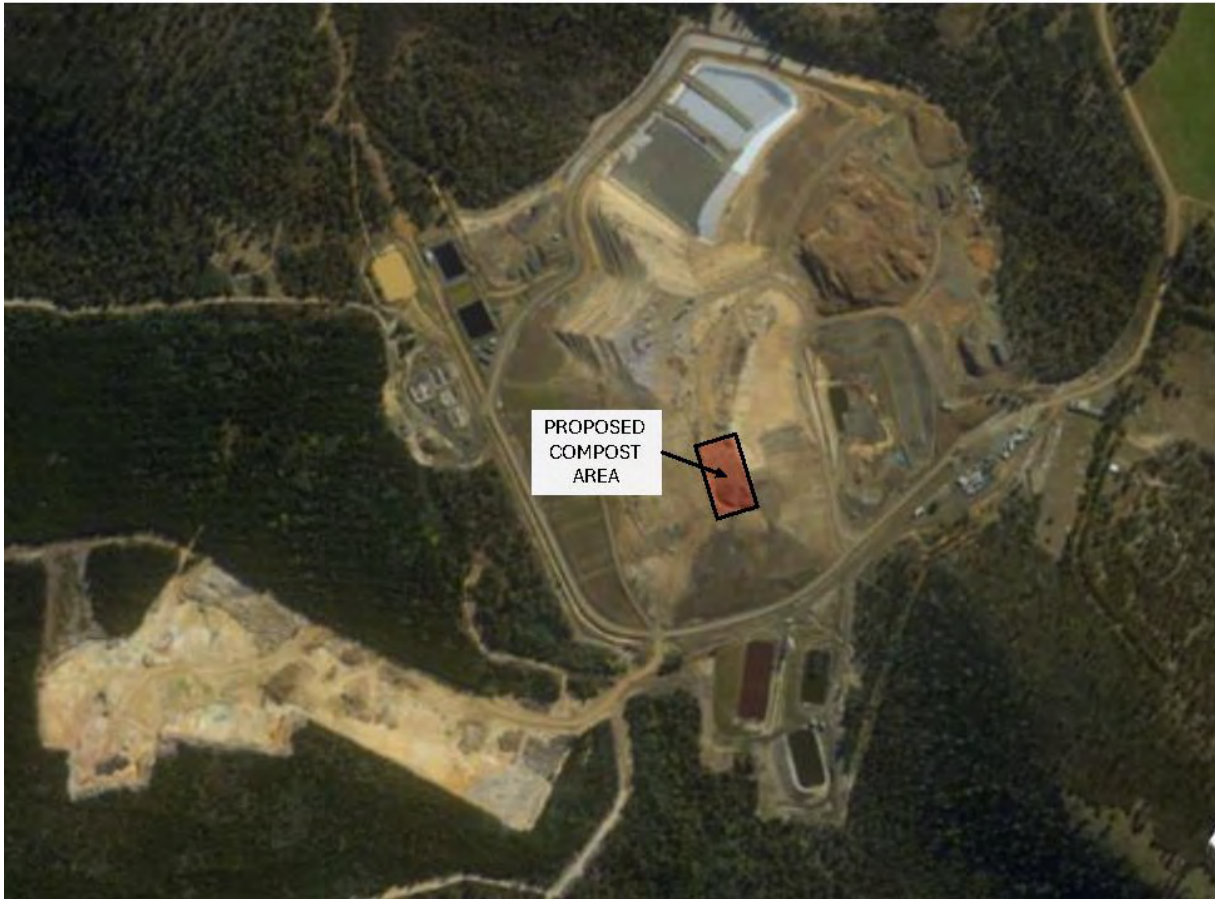
Figure 3 Location of interim facility, atop B cell with interim capping.
