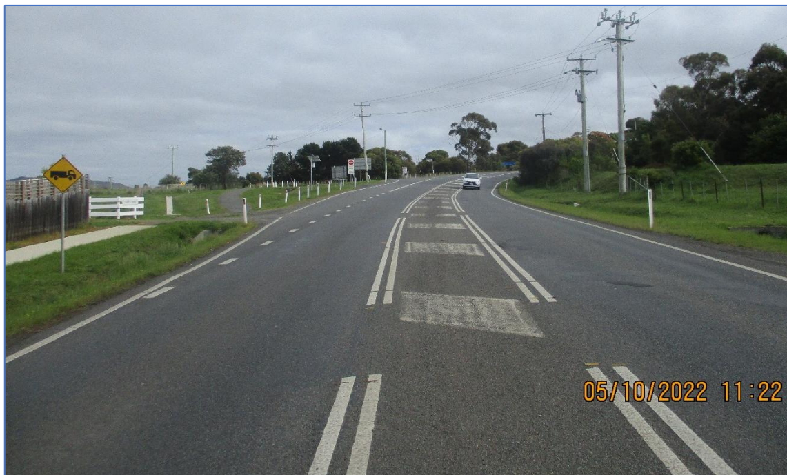
Photograph 5.1 – Tasman Highway standard
