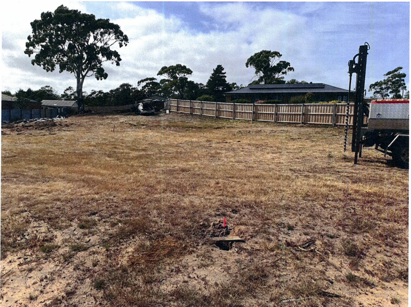
Plate 4 – Test Hole #5 - looking to the east.
