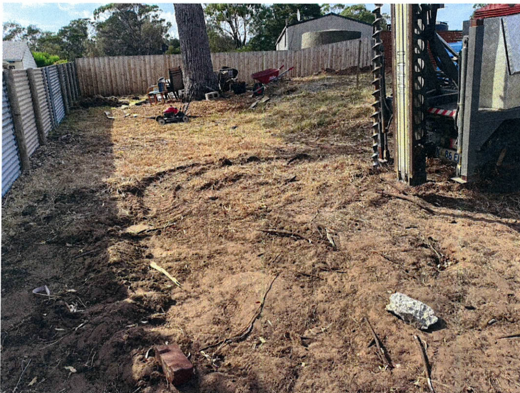
Plate 2 – Test Hole #2 - House site test hole - looking to the southeast.
