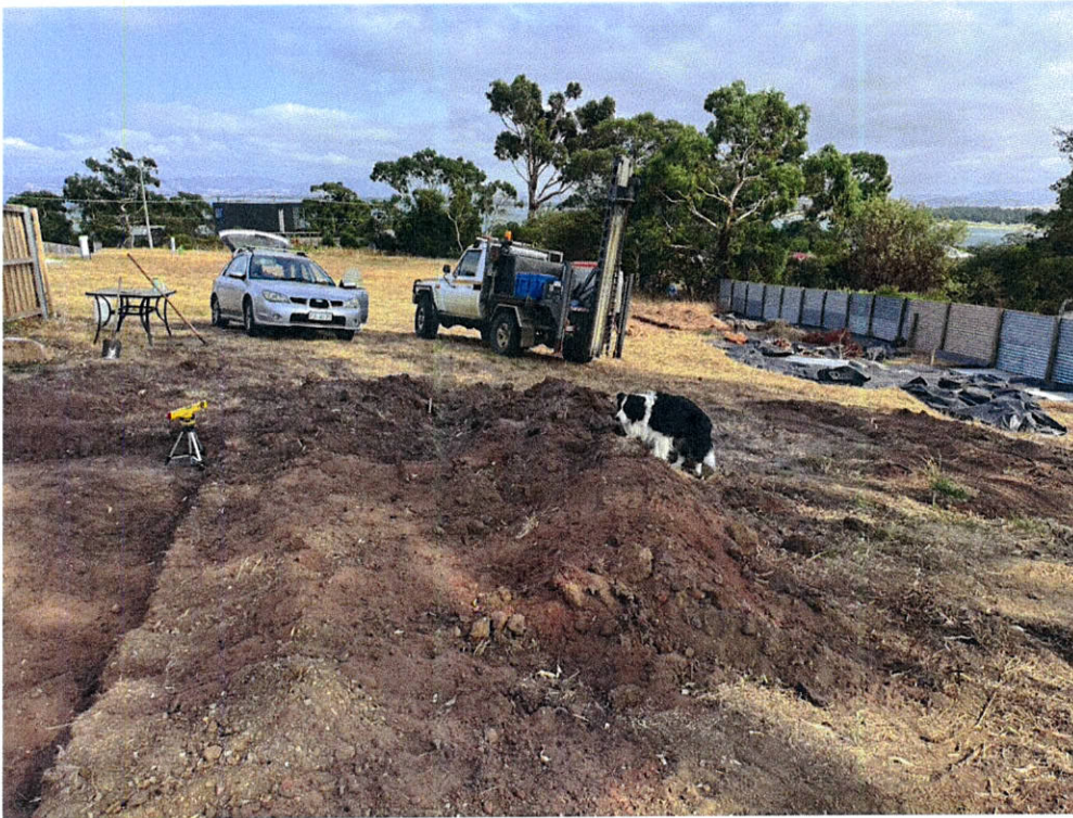
Plate 3 – Test Hole #3 - House site test hole - looking to the northwest.
