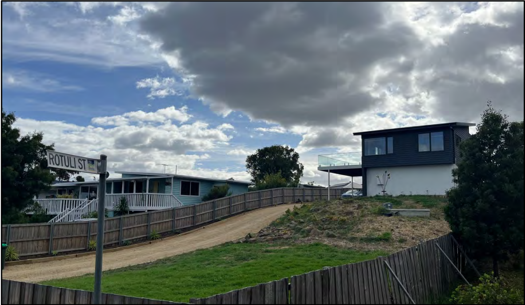
Figure 8. 124 Bally Park Road (right) relative to 122 Bally Park Road (left). Both of these properties adjoin the site.
