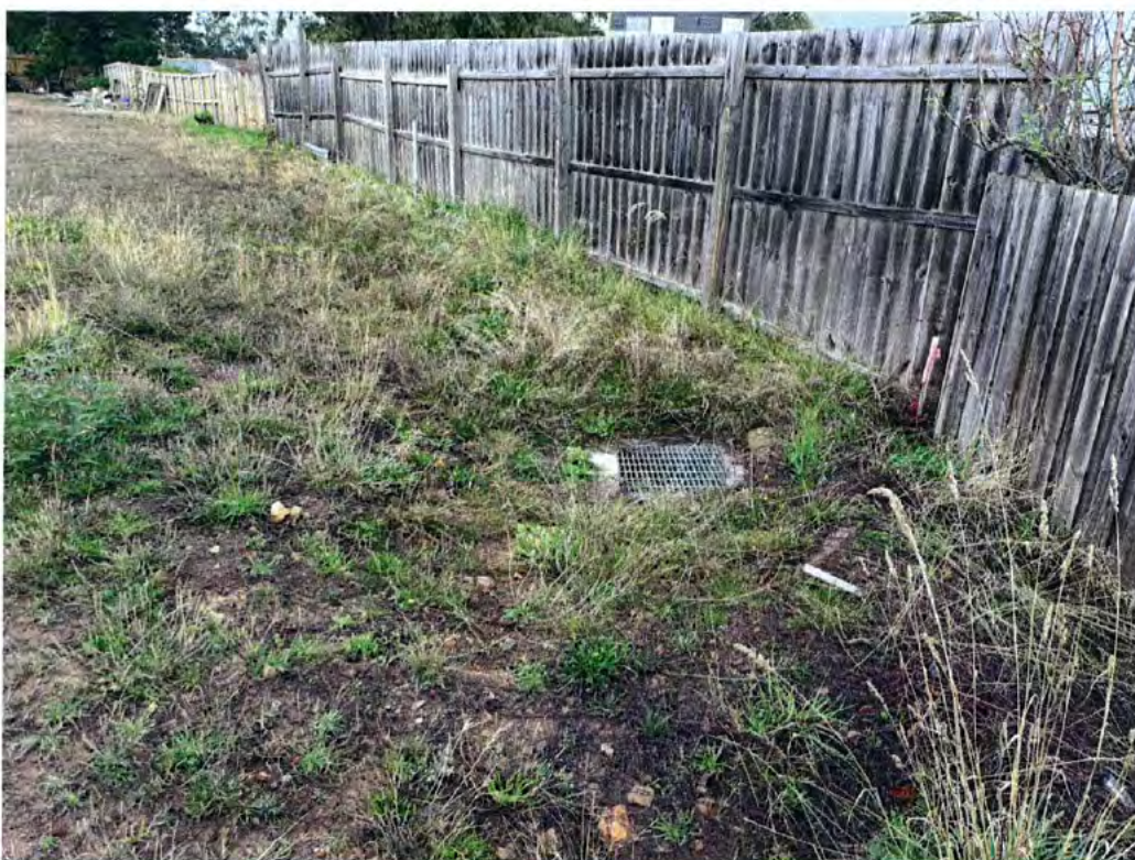
Plate 2 – Stormwater drain on the western side of the property - looking up-slope to the south.
