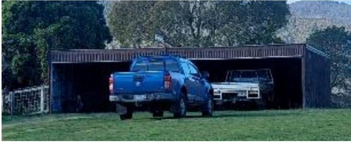
Figure 18: the garage (from the Bushfire Report). Headroom at the entrance is 2.05m.
