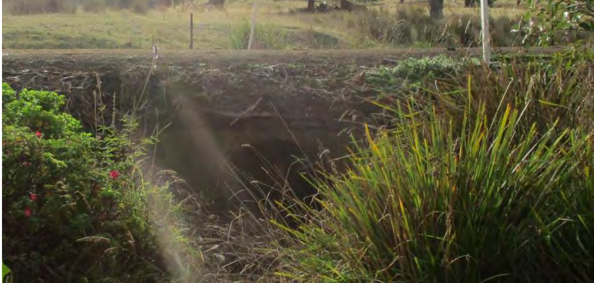
Photograph 5.3C – Pipe culvert 185 metres south of Fulham Road
