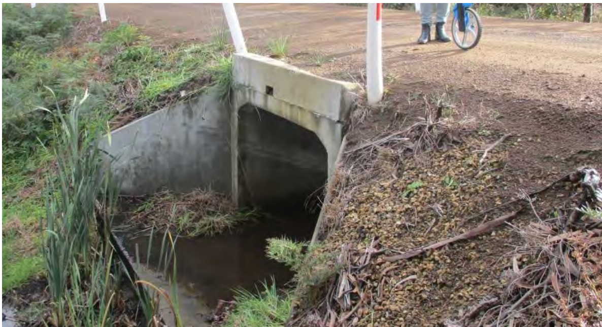
Photograph 5.3D – Box culvert 260 metres south of Fulham Road
