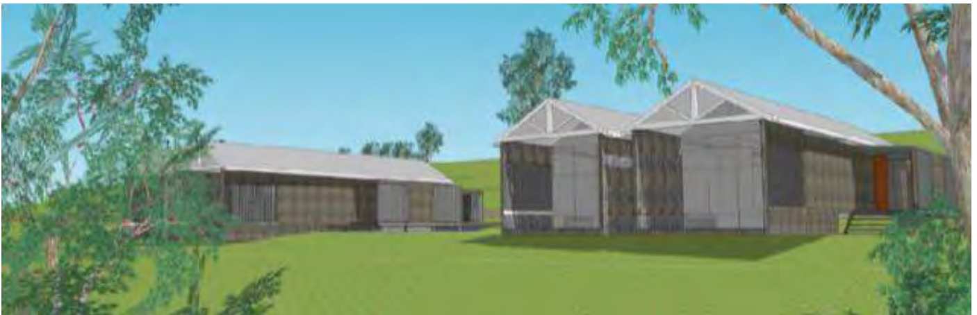
Image 18: Southern view of Boat Houses (Type D cabins)
