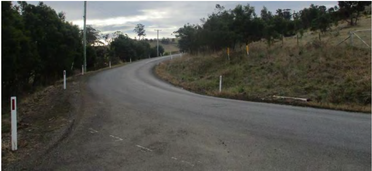
Photograph 5.5A – Available sight distance to the left (120 metres)
