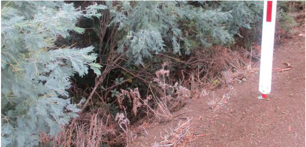
Photograph 5.3E – Pipe culvert located 420 metres south of Fulham Road
