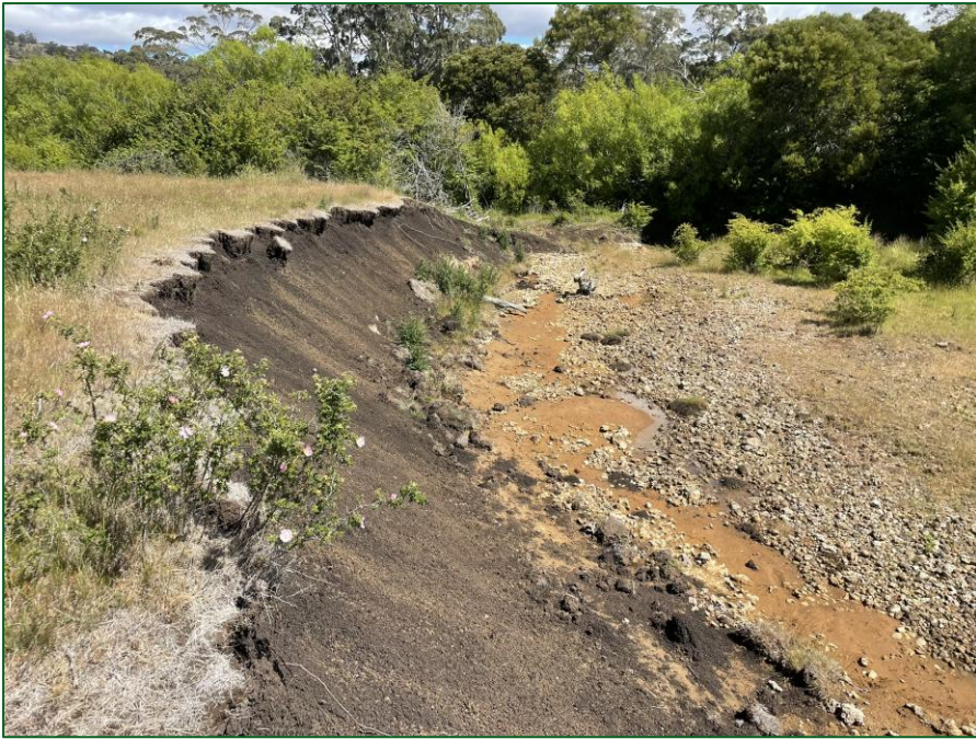
Figure 14 Black cracking clay loam soil graduating to sandy alluvial soil topsoil over a clay subsoil on stream banks and river flats. Taken at site assessment 22/12/2025.
